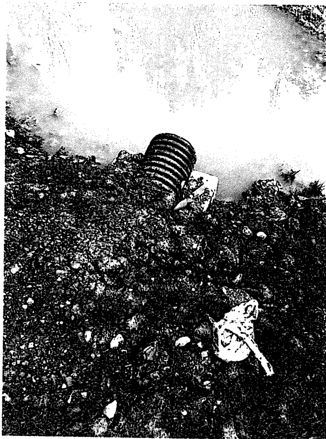
12" INLET AND HALF CONCRETE HEADWALL
