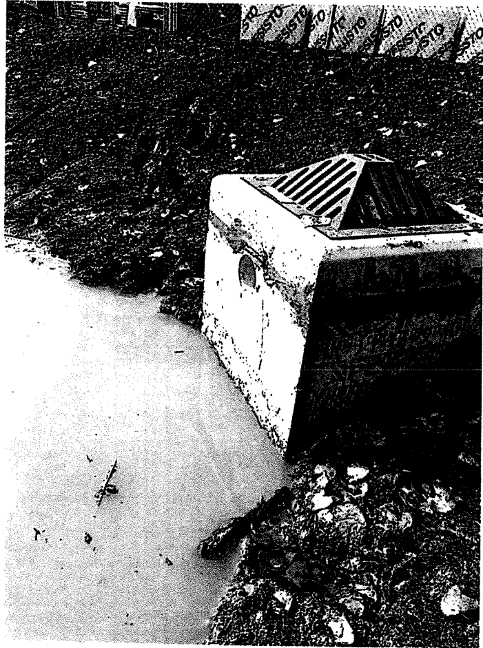
OUTLET STRUCTURE EXTERIOR
