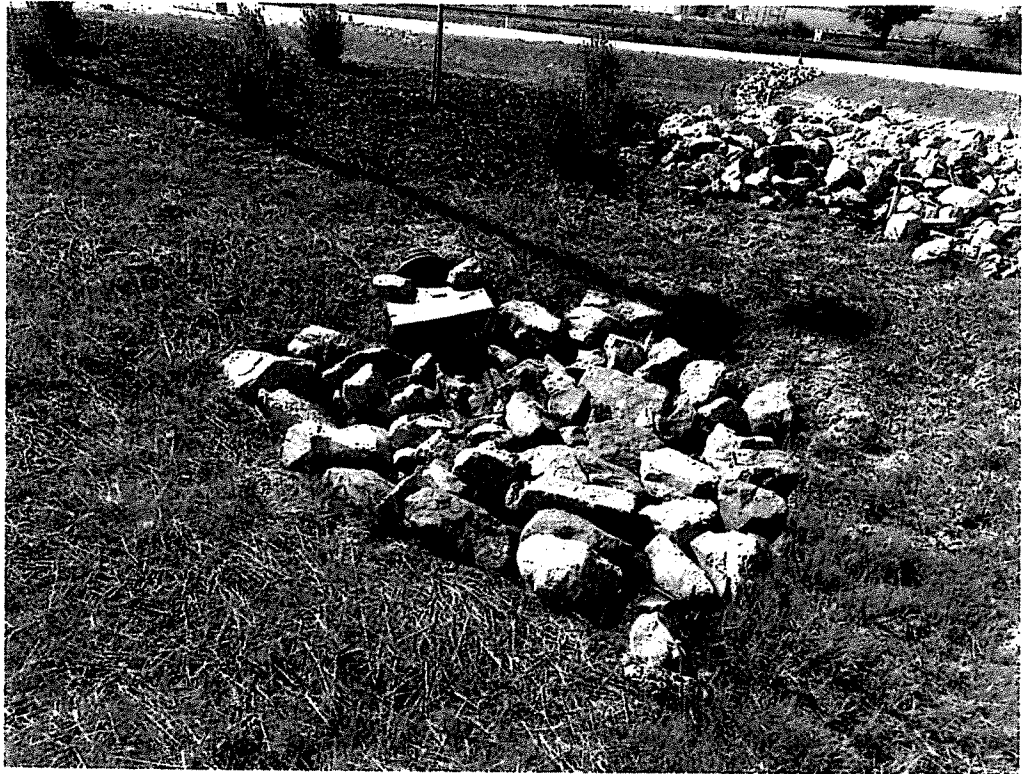
Existing 18" Storm – Downstream End
