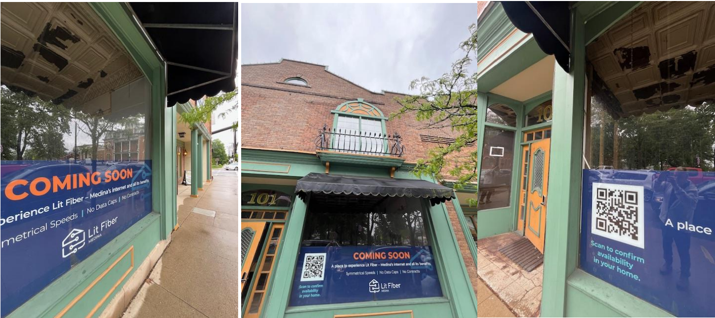
First Floor Window Replacement -
